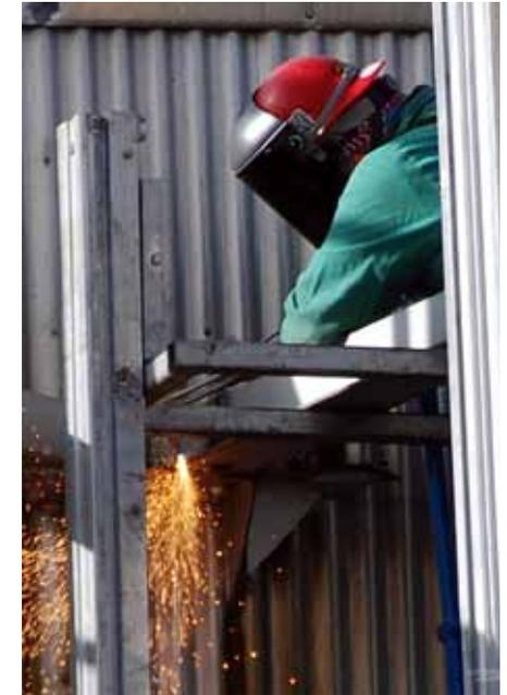
*A worker cuts the metal beam bracing one of the MFC boiler stacks that were removed during facility upgrades. Removal of the boiler stacks was visible evidence of INL's commitment to reduce greenhouse gas emissions and reduce water waste.*
