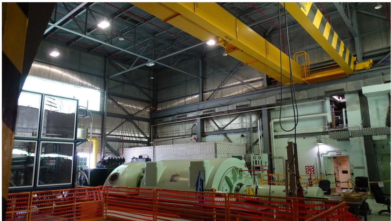
Figure 11. Present overview of third floor (INL CRMO 2024).
