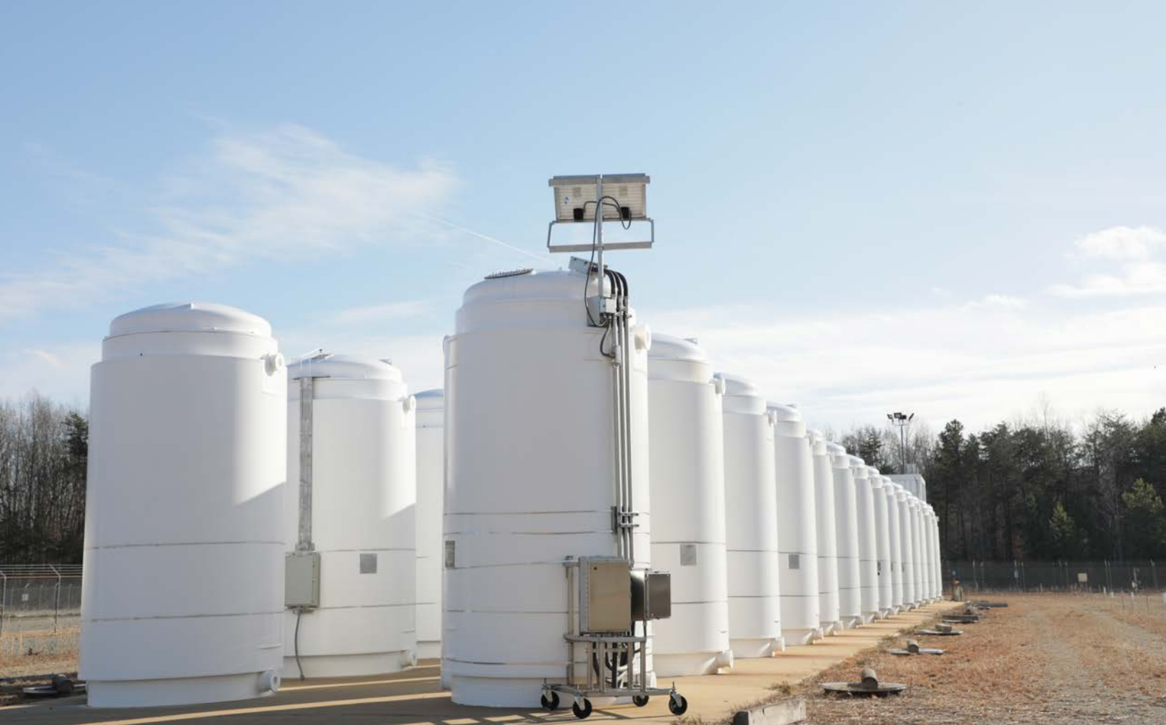
Dry storage systems and the High Burnup Research Cask at the North Anna Power Station.
