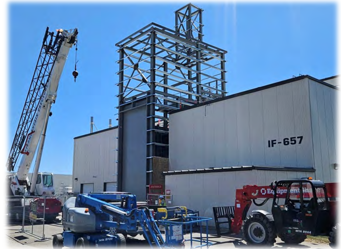
Figure. IEDF during infrastructure upgrade.
