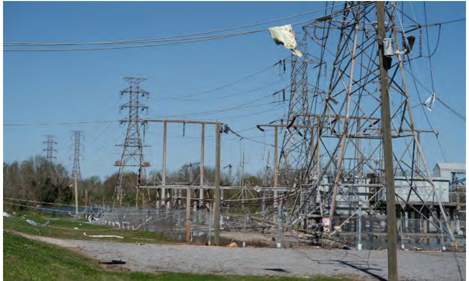
Figure 5: Storm-DEPART has been used by the Louisiana-based utility Entergy to improve their response to two hurricanes.
