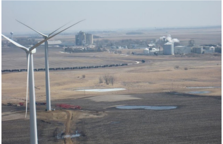
Iowa Lakes Wind Farm – Superior Site, supporting a local ethanol plant [1].
