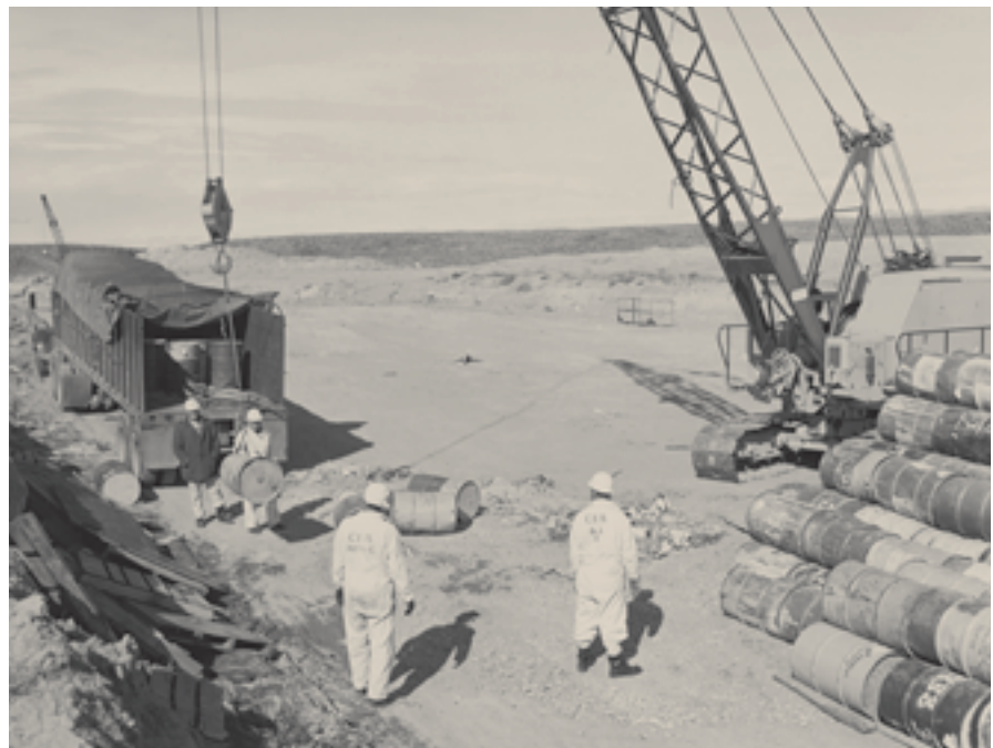
A crane helps workers unload Rocky Flats barrels in 1961.
