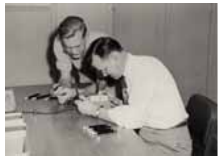
Calibration technicians check ionization chambers of a minometer. Site employees wore them in their pockets. The devices were checked daily for possible exposure to radiation.
