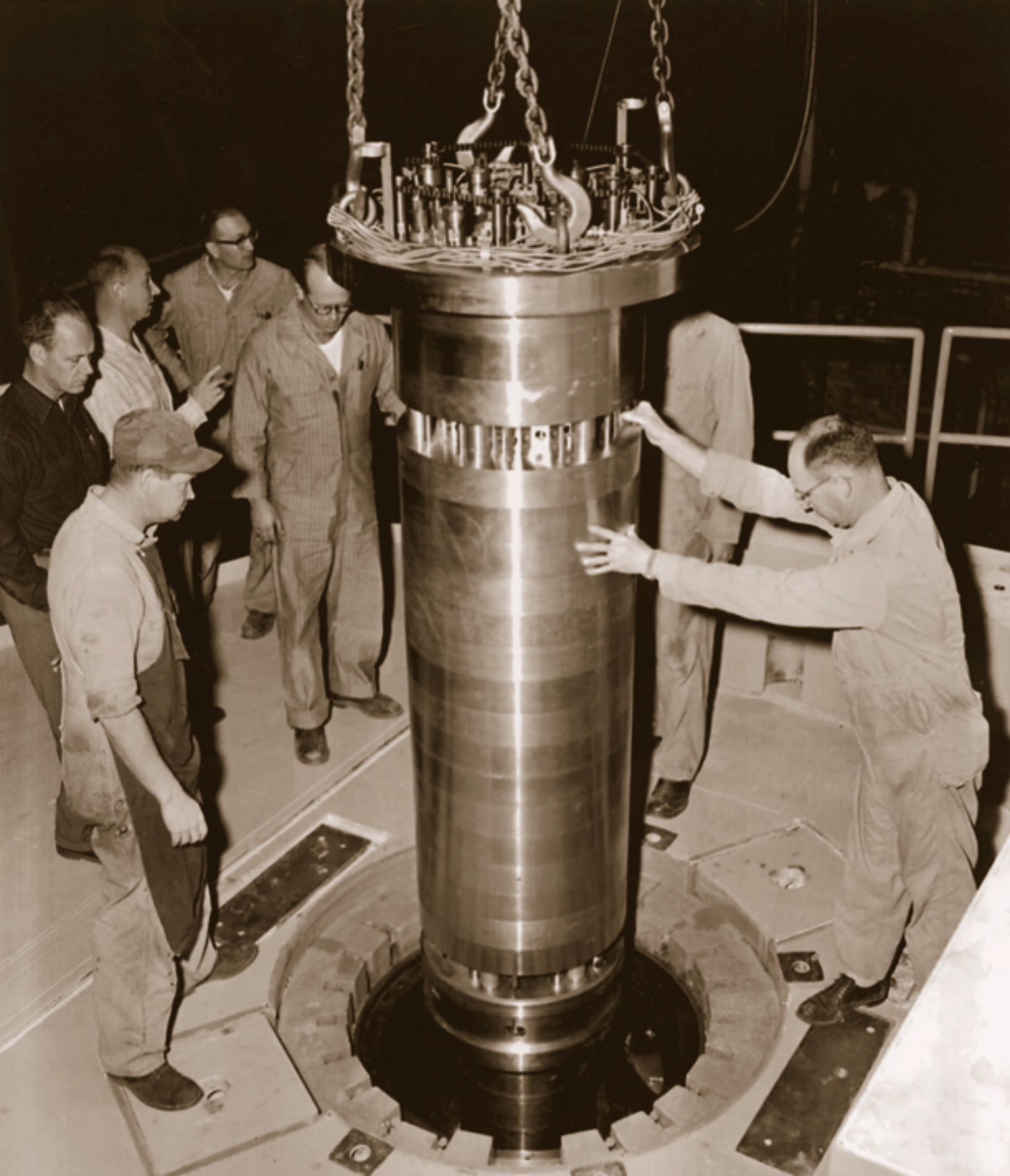
Installing the reactor vessel into EBR-I.
