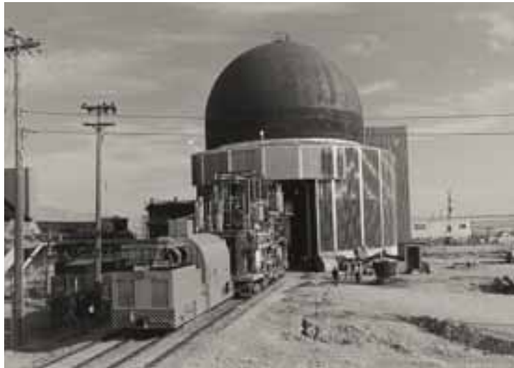
LOFT reactor being moved into containment vessel.
