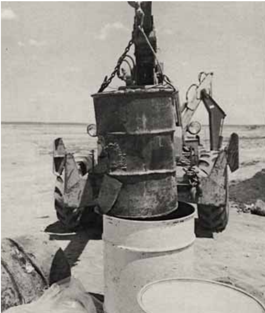
Damaged waste barrels retrieved in the 1970s were sometimes placed in "overpack" barrels.
