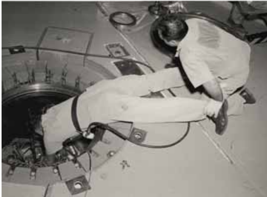
Teamwork inside the NRTS duplicated the outside teamwork among NRTS supporters. Here, technicians work over the core of EBR-I.
