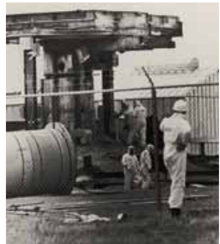
Right. Foundation piers and gravel were all that remained by 1962. Debris went to a special SL-1 burial ground. Below. Dismantling the SL-1 foundation piers required the use of shaped charges. Here crew wires caps to charges.
