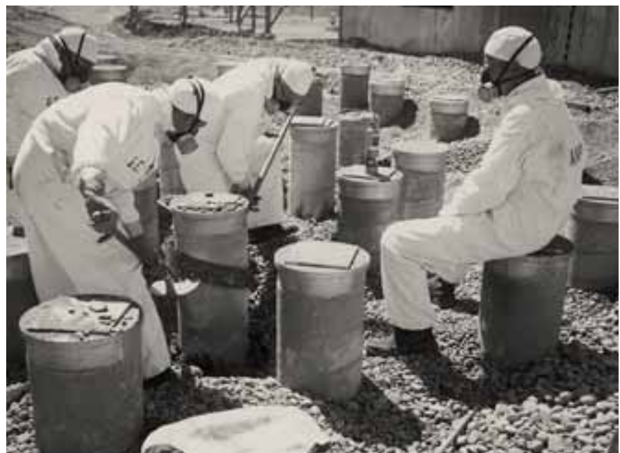
Right. Foundation piers and gravel were all that remained by 1962. Debris went to a special SL-1 burial ground. Below. Dismantling the SL-1 foundation piers required the use of shaped charges. Here crew wires caps to charges.
