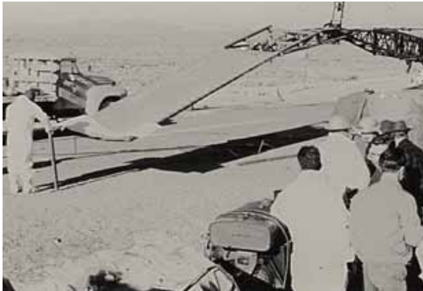
The stretcher rig. Crews practiced before the rig was inserted into the reactor building to collect the body of the third man.
