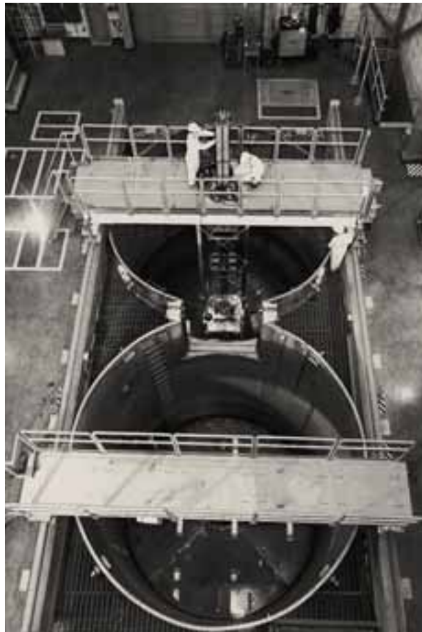
Twin pools of the SPERT-IV reactor facility, under construction in 1961. The men on the bridge stand over the reactor pool. The other pool was used mainly to store fuel, but added to the general flexibility of operations.
