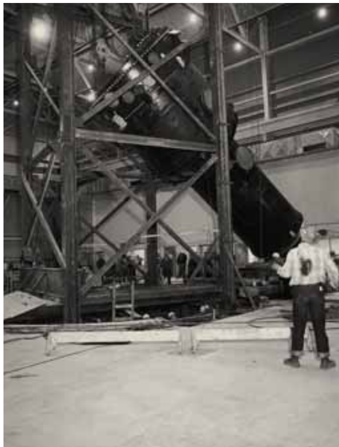
ETR reactor vessel being raised to vertical position during construction in 1956.
