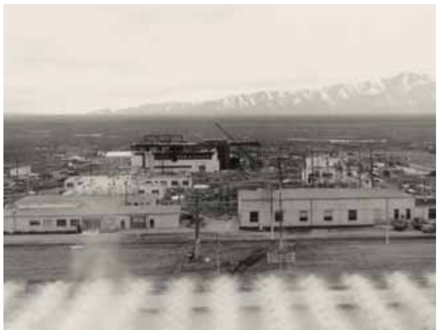
A1W under construction. Photo, circa 1956, shows S1W spray pond in foreground.
