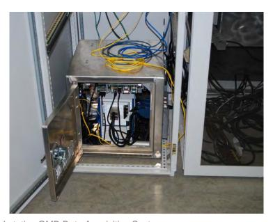
Figure 2. INL Typical Substation GMD Data Acquisition System.
