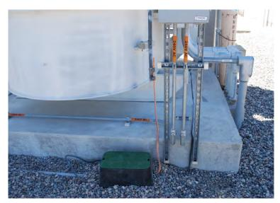
Figure 1. INL Typical INL Transformer - GMD Ground Current Measurement.
