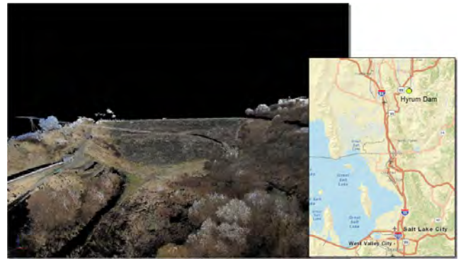
FIGURE 1. 3-D point cloud data and location map of Hyrum dam.
