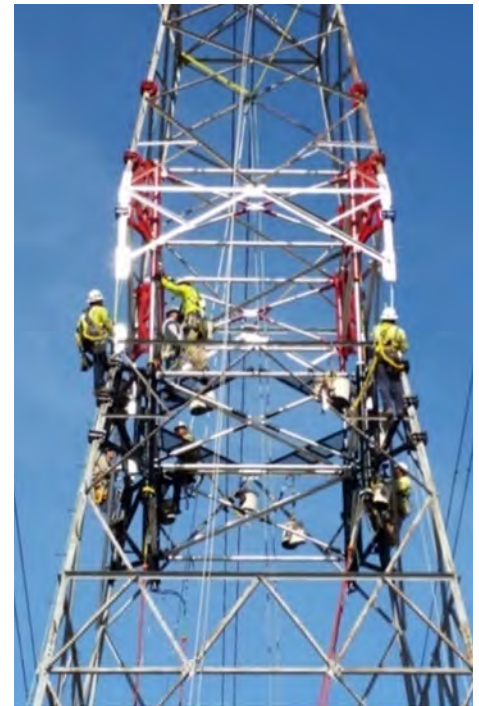
Figure 2-11. Linemen raising the height of a tower.
