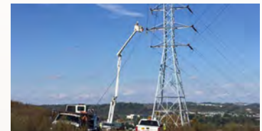
Figure A-38. Tower reconductoring.
