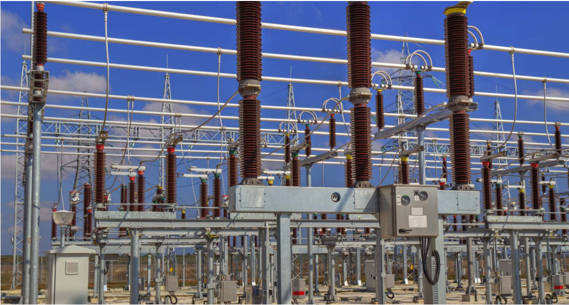
Figure 2. Substation circuit breaker used to modify system topology.
