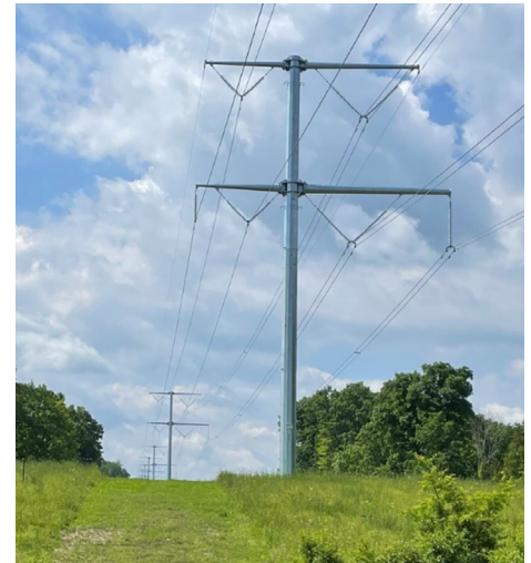
Figure 2-17. A double circuit rebuild for the New Your Energy Solution project with the 115 kV circuit on the left side of the tower and the 345 kV circuit on the right side of the tower.
