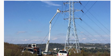
Figure A-38. Tower reconductoring.
