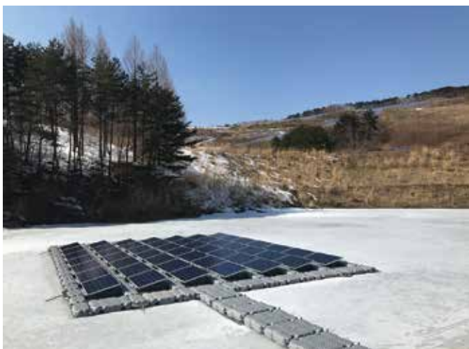
FIGURE 1.9. Deployment of FPV in freezing conditions in Japan (left) and China (right)
