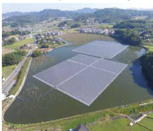
FIGURE 6.7. Examples of SMCC’s FPV systems in Japan
