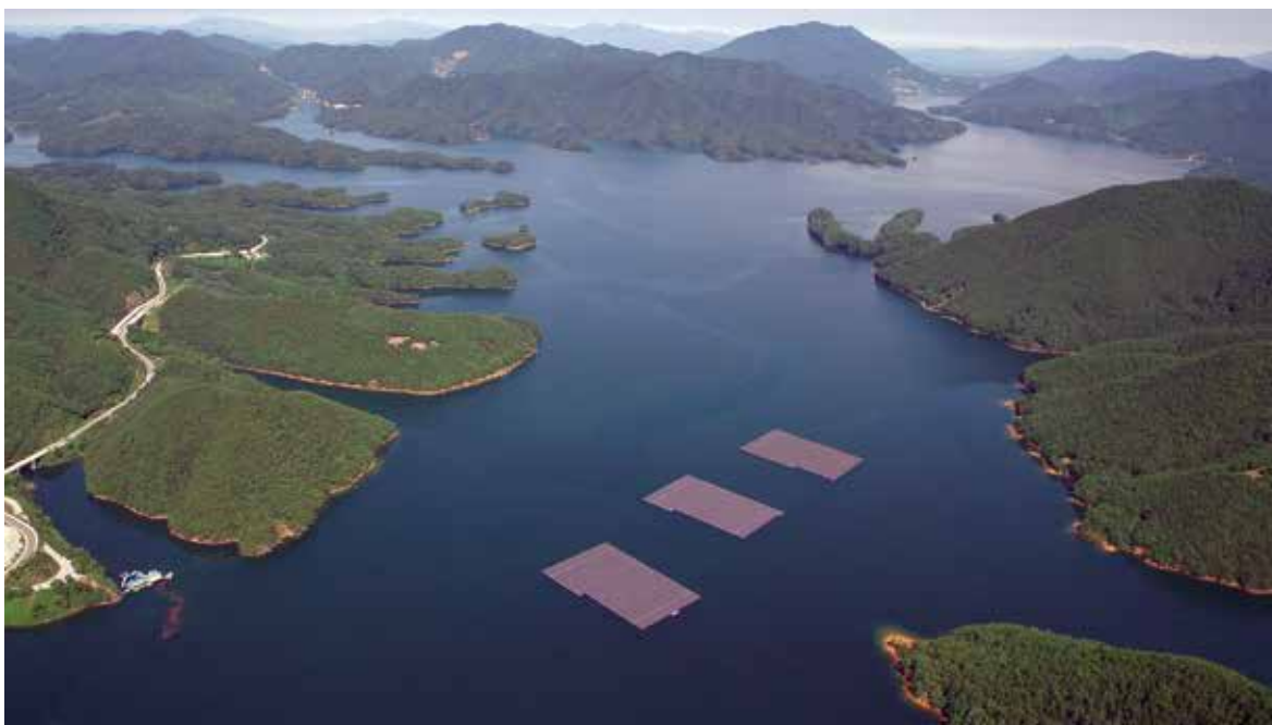
FIGURE 3.11. FPV installation (with a capacity of 3 MWp) Cheongpung Lake, Chungju Dam in Korea
