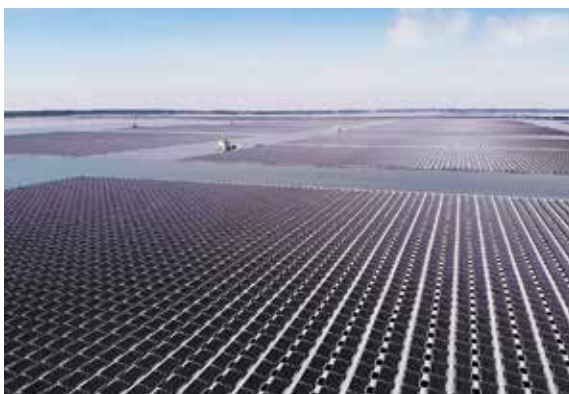
Source: © Sungrow. Note: kWp = kilowatt-peak; MWp = megawatt-peak.
