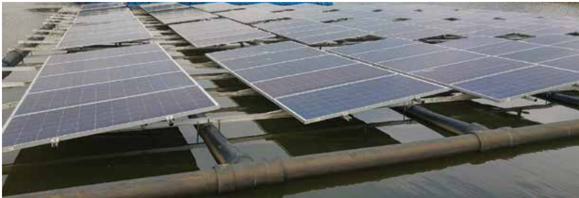
FIGURE 2.7. Various designs using metal frames and pipes to support PV panels, 4C Solar (top) and Koinè Multimedia (bottom)
