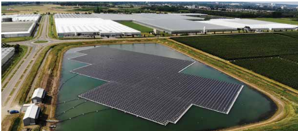
FIGURE 3.7. FPV installation (with a capacity of 1.85 MW) in Azalealaan, Netherlands
