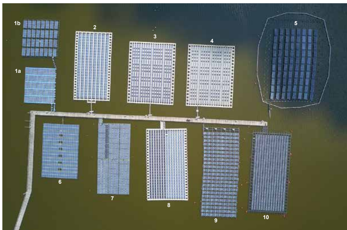
FIGURE 3.10. SERIS FPV testbed (with a 1 MWp capacity) at the Tengeh Reservoir in Singapore
