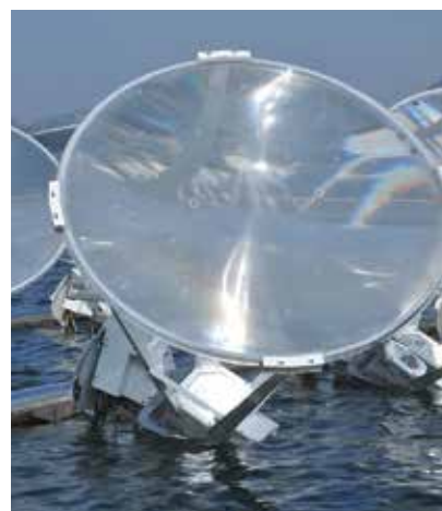
FIGURE 2.19. Sunengy's Liquid Solar Array with dual-axis tracking and concentrators (left), detail of the collector with lens concentrator (right), Whalvan Hydroelectric Dam, Lonavala, Maharashtra, India
