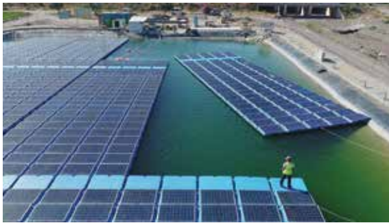
FIGURE 1.7. FPV system for covering of entire reservoir surface to reduce water evaporation
