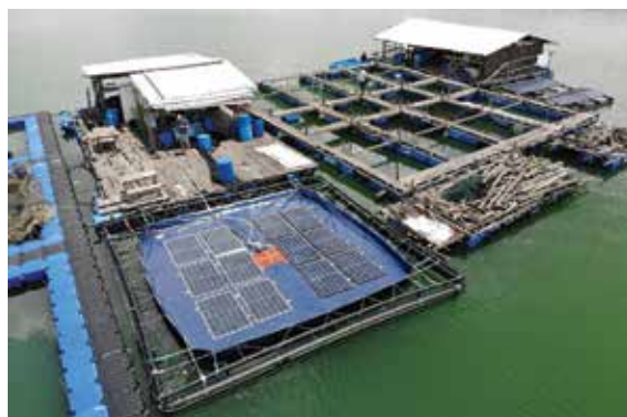
FIGURE 1.6. Floating solar for fish farming in Singapore
