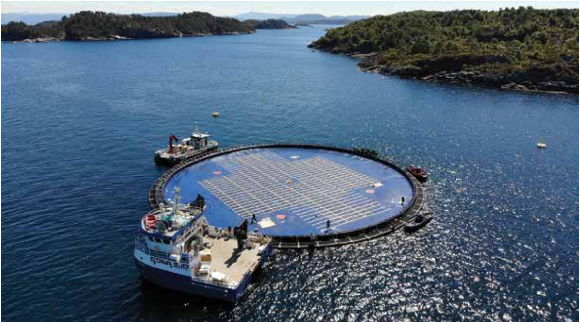
FIGURE 2.24. Ocean Sun’s offshore floating platform in Norway, with membrane to hold PV panels
