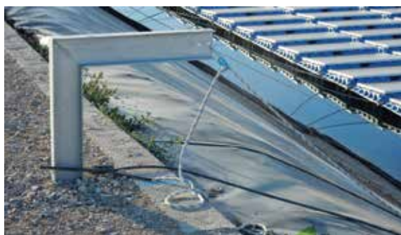
FIGURE 2.12. Bank anchoring example
