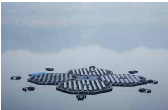
FIGURE 2.16. The 100 kW tracking FPV plant at Hapcheon Dam, Korea
