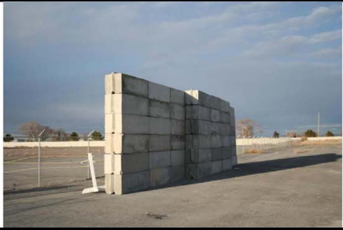
Figure A-7. Example of beam stops assembled using concrete blocks; this picture shows a typical beam stop for the Varitron-III shielding. Each block is 2' thick, 2'tall and 6' long. The delivery and placement of shield blocks require forklifts and semi-trucks. The movement of a large number of blocks usually only happens once every few year.
