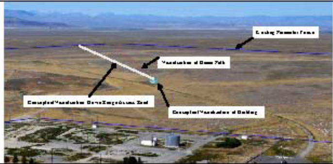
Figure A-11. Visualization of SOX Range with building, down-range road, and possible beam path and with TAN/TSF in foreground
