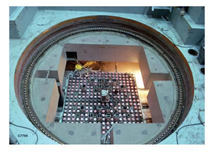
Figure 1. Photograph of the top of the TREAT reactor at the INL showing the circular top of the fuel elements supported by the rectangular fuel plate; the experiments are usually placed in the center, of the reactor. The rotating shield plug is not present in the picture.
