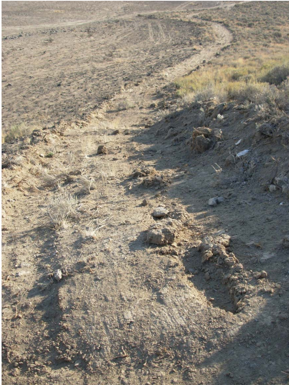
Very steep side hill that has extensive damage from dozer.
