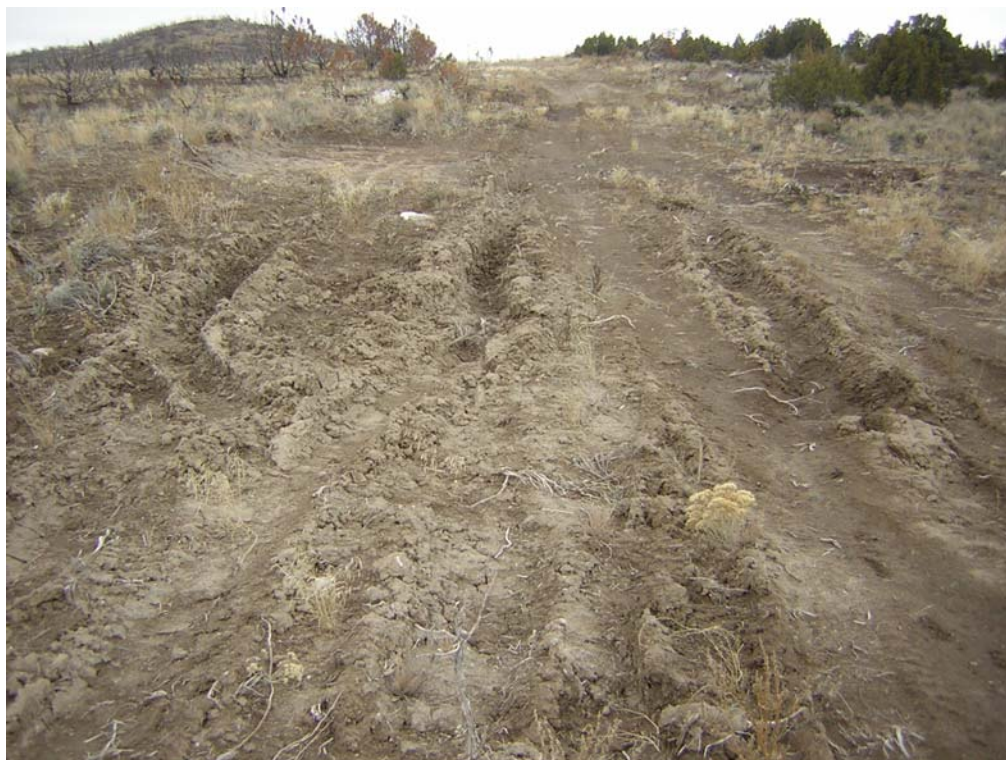
Figure 8. Containment line on Twin Buttes Fire showing ruts created by vehicles during wet weather.
