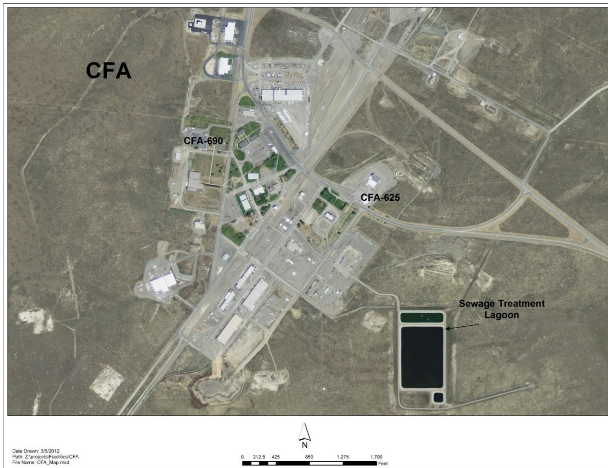
Figure B-3. Location of selected facilities at CFA.
