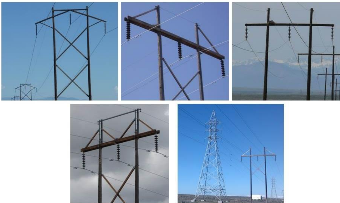
Figure 4-3. Transmission pole structures used as nest substrates by ravens in 2016. From Left to Right:(Top) Sloped H, Closed H-Cable, Open H, (Bottom) Hybrid, Lattice.
