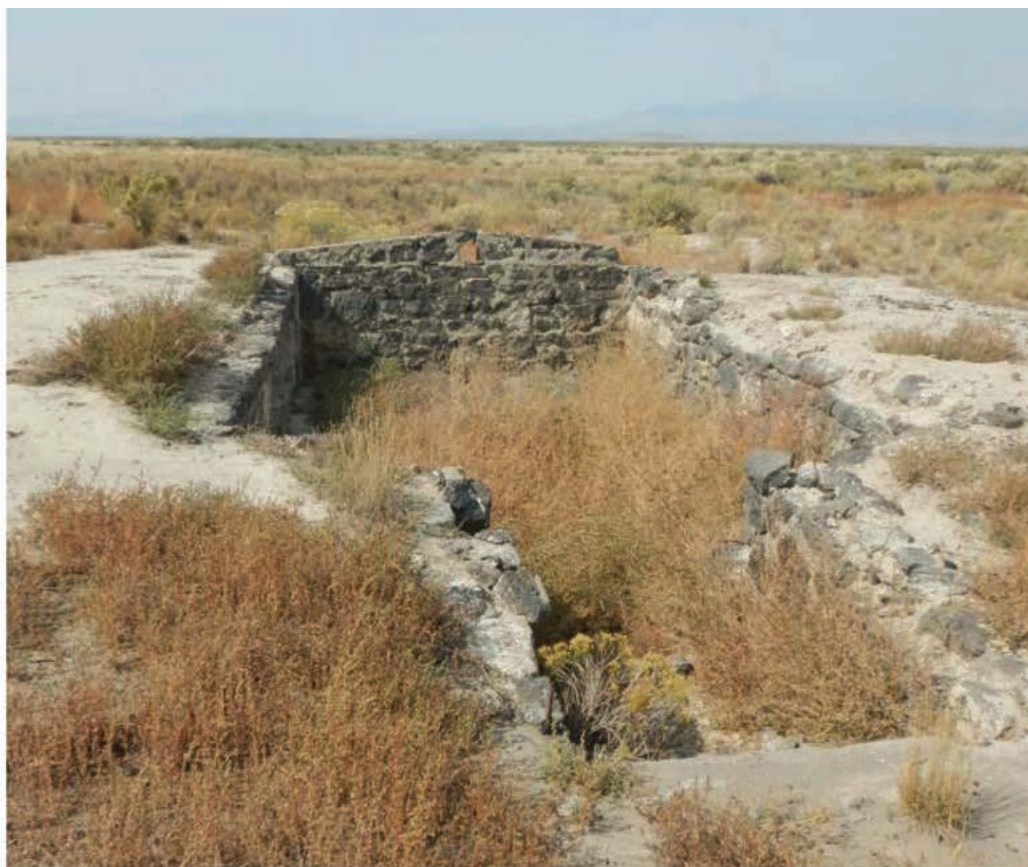
Figure B-3. Basalt Foundation of Homestead Located in the Second Owsley Project. The Homestead is Surrounded by Foundations for Other Structures, Field Levees, and Ditches That Cover an Entire Public Land Survey System Section North of the Main Canal.
