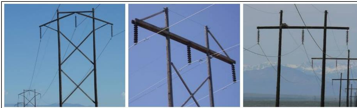
Figure 4-3. Transmission pole structures used as nest substrates by ravens in 2015. From Left to Right: Sloped H, Closed H-Cable, and Open H.
