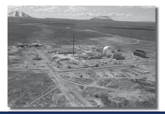
Header Photo Description: The investigation of fast neutron breeding reactors began at Experimental Breeder Reactor I or EBR-I in 1950. Beginning in 1964 the work was continued inside the silver-domed containment shell at EBR-II. The EBR-II reactor operated with an ahead-of-its-time closed fuel cycle, efficiently providing electricity for most INL Site operations for a number of years.
