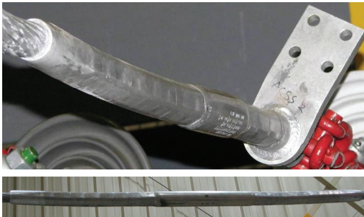
Figure 2-50. Southwire ACSS conductor with AFL Global two-stage compression connector installed
