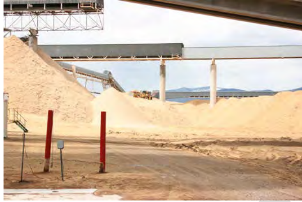
Figure 2-39. Enclosed belt conveyor at Smurfit Stone paper mill, Montana (Photo credit: D. Brad Blackwelder, INL).
