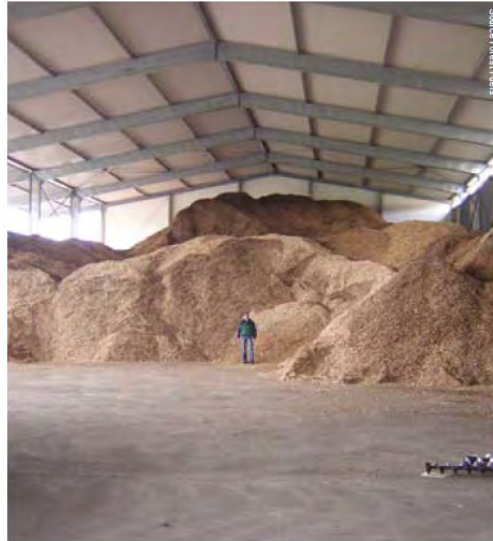
Figure C-1. Large-scale enclosed chip fuel storage (Regensw Sustainable Energy Agency 2008).
