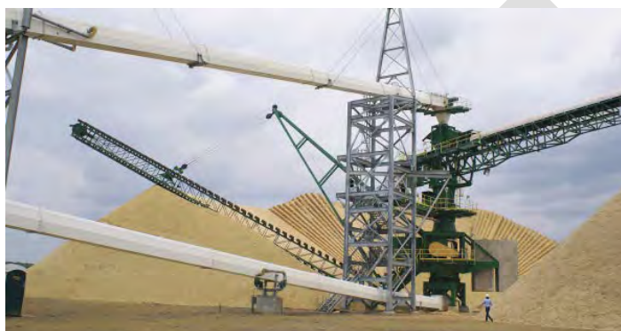
Figure 2-40. Bruks circular stacker reclaimer at the Green Circle pellet mill in Cottondale Florida. The contained, white conveyor at the top drops clean chips on the green conveyor going to the right. Simultaneously, the bucket reclaimer is pulling chips off the pile on the left and depositing them on the lower, contained conveyor, which is taking them to the pelleting facility (Photo credit: Bruks 2010).
