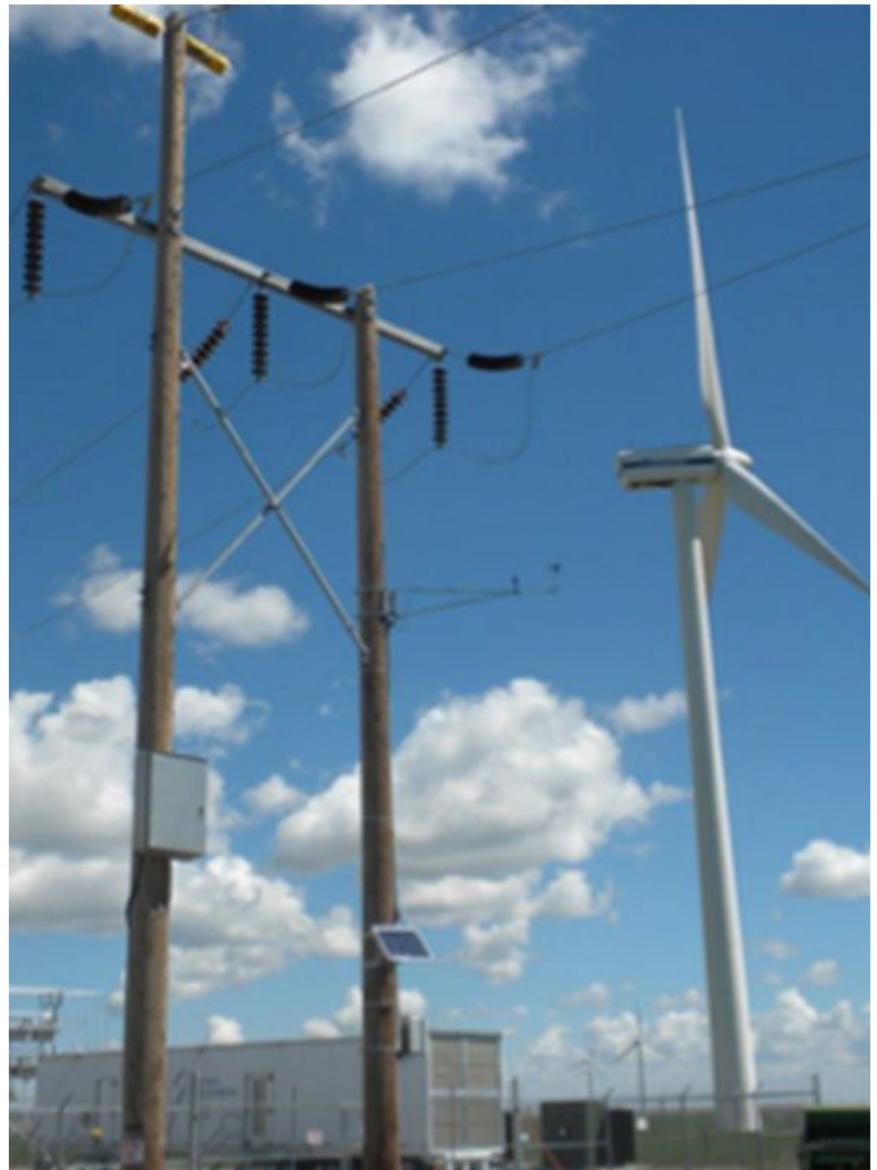
Weather station configured on an electric utility transmission line structure.
