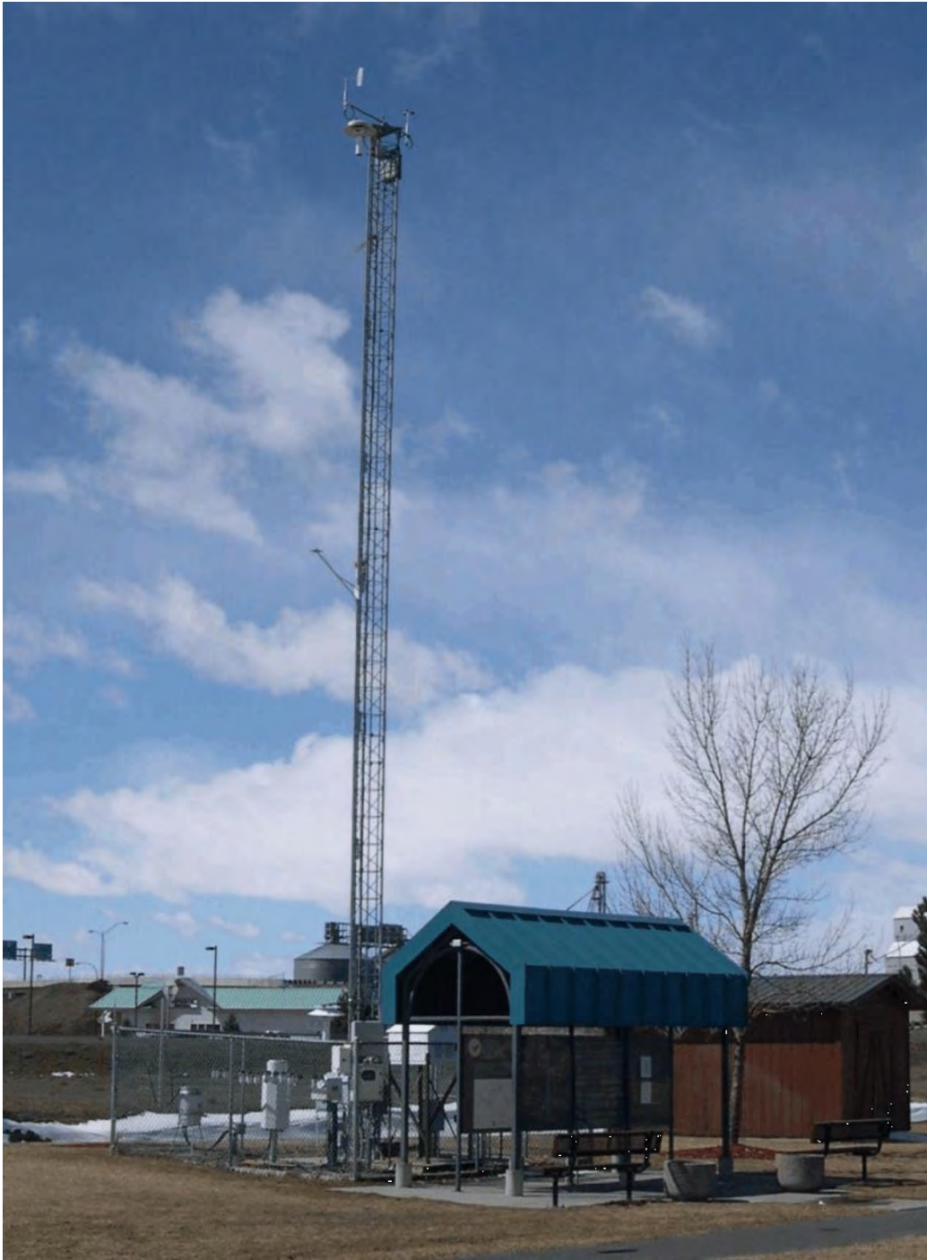
Figure 3. Example NOAA/INL Mesonet Station Layout and Community Monitoring Station Kiosk (foreground) on the Idaho Falls Greenbelt at the John’s Hole Bridge and Forebay.
