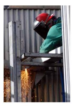
A worker cuts the metal beam bracing one of the MFC boiler stacks that were removed during facility upgrades. Removal of the boiler stacks was visible evidence of INL's commitment to reduce greenhouse gas emissions and reduce water waste.
